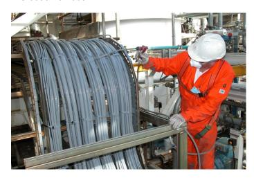
Avicoat is often used in confined spaces in underground and marine / shipping situations where burning cables can create hazards from smoke, toxicity and unnecessary power failure.
